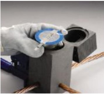
Step 1 Insert CADWELD PLUS package into mold.
