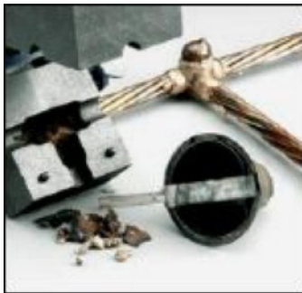
Step 4 Open the mold and remove the expanded steel cup - no special disposal required.
